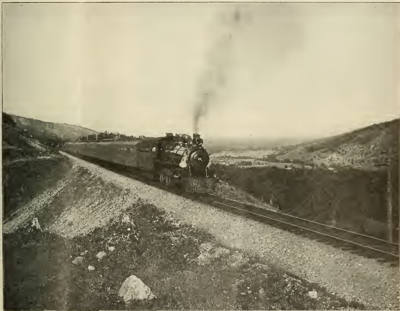
THE MARITIME EXPRESS ON THE INTERCOLONIAL RAILWAY OF CANADA.
